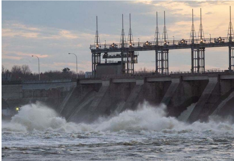
Carillon Dam located in the southern portion of the Ottawa River on April 25, 2019
