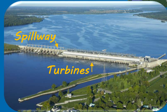
Run-Of-River Generating Station
