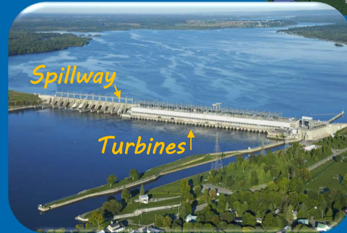
Run-Of-River Generating Station
