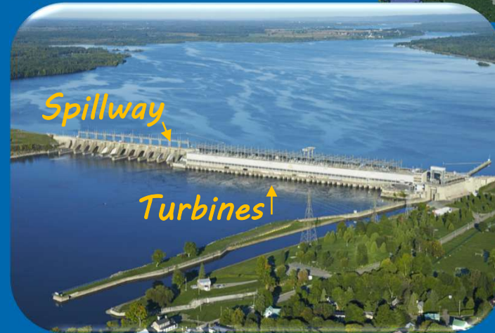
Run-Of-River Generating Station
